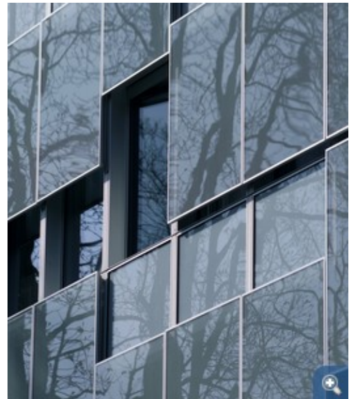
Detail of the new facade with movable parapet elements made of glass and metal mesh, which provide sun protection that can be controlled room-wise.
