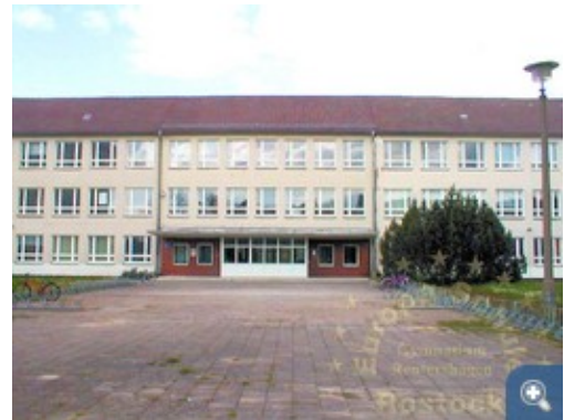
Entrance area of the existing school before refurbishment
