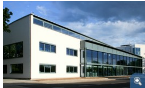
The west facade of the printing building in Karlsruhe after being refurbished and extended. © Patrick Beuchert, www.patrick-beuchert.de
