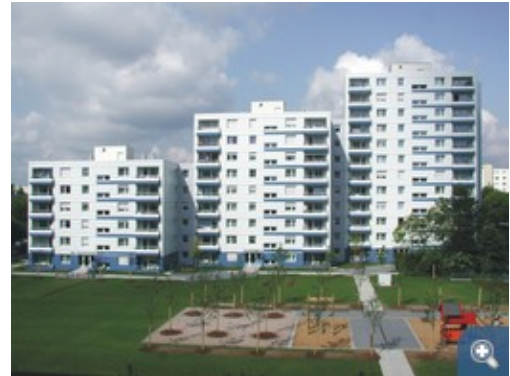
After refurbishment, the high-rise residential complex is barely recognisable. Alongside the energy-related advantages, a considerable aesthetic improvement was achieved.
