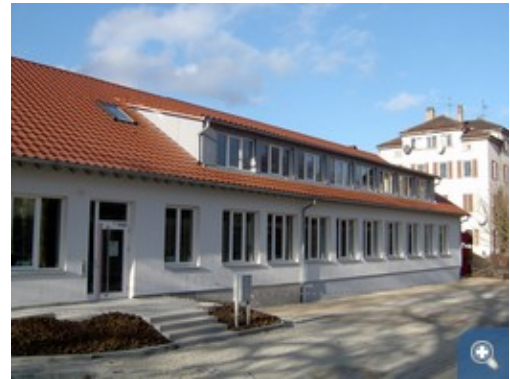
East elevation of the refurbished building on the site of the former Thiepval barracks © ebök, Tübingen
