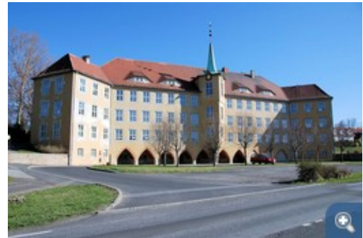
The school in Olbersdorf before refurbishment: Once refurbished, the building from the Weimar period is intended to achieve the so-called 3-litre house standard.
