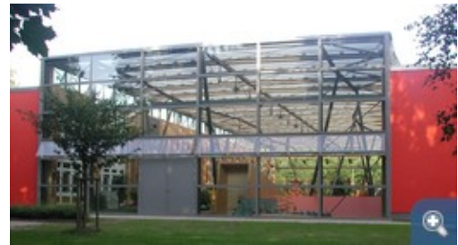
A thermal insulation composite system with vacuum insulation panels was installed on the western end wall facade.
