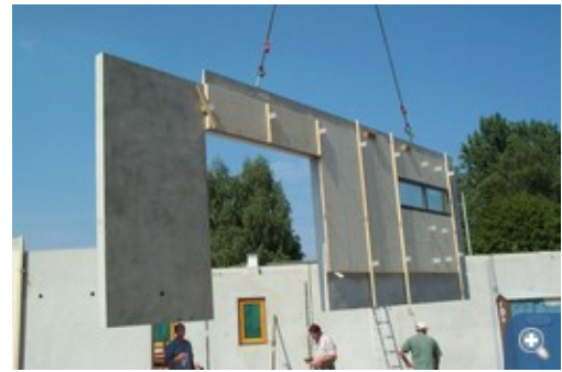
The application of vacuum insulation panels under construction.
