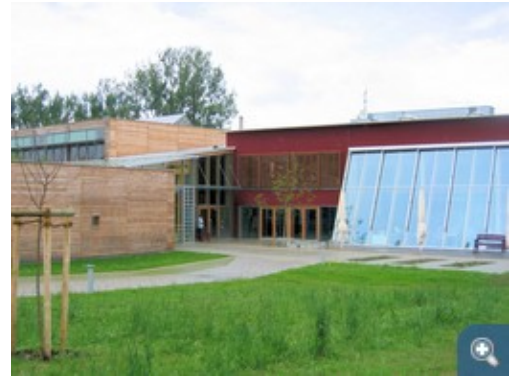
Wood and glass define the appearance of the workshop for disabled people in Lindenberg. © Lichtblau Architekten
