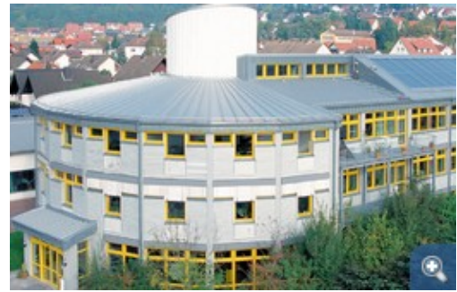
The first office building built in Europe according to the passive-house philosophy was also one of the first EnBau model projects – the administration building of a medium-sized solar technology company in Cölbe.
