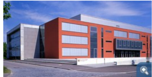
Daytime view of the vocational school in Biberach, as seen from Leipziger Strasse.
