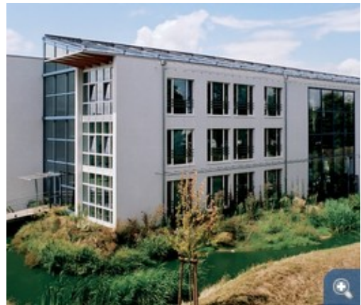
The SurTec GmbH building viewed from the south: the administration block is shown. Behind this is the atrium, which connects administration with the chemical laboratory.
