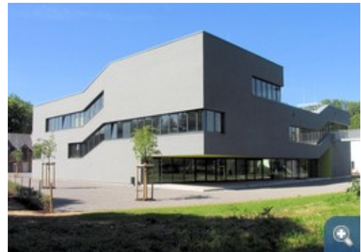
The Science College shortly after the inauguration of the building on 27 June 2009.
