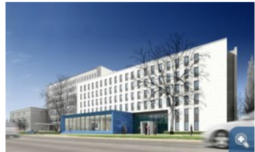
The new Regionshaus building in Hanover. Visualisation from the perspective of Hildesheimer Strasse.
