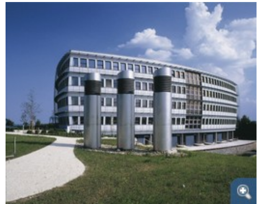
A general view of the Energon building. The towers in the front belong to the ventilation system. © Software AG Stiftung
