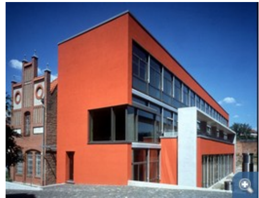
The glazed south facade of the ZUB Kassel, allows an ideal use of daylight. © ZUB Kassel
